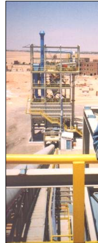
Dolomite & limestone crushing and ensiling
