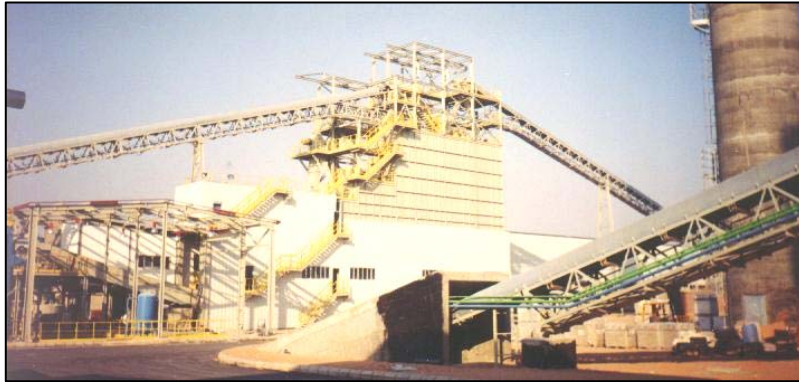
Batch plant: Main silo and weighing building
